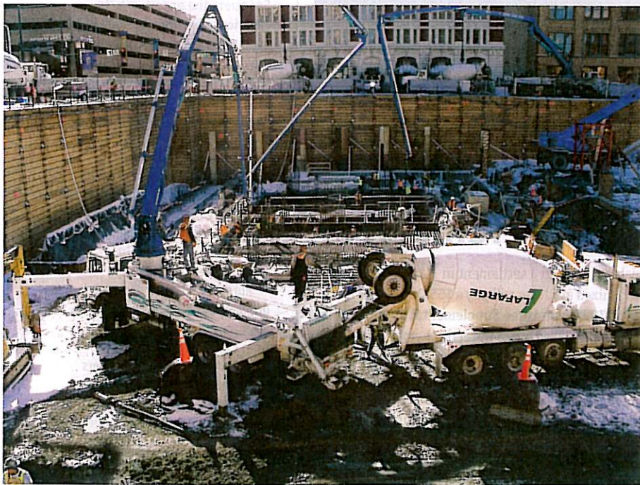
PHOTOS: Rocky Mountain Precast/Swinerton Builders
